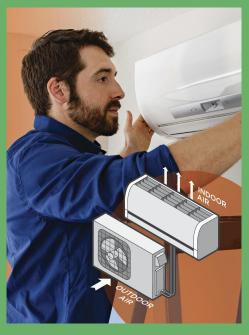
mini-split systems have two main components—an outdoor compressor and an indoor air-handling unit(s). A narrow conduit links the indoor unit(s) to the outdoor compressor.
